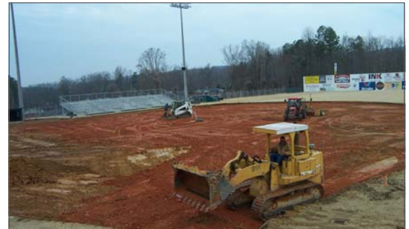
Excavation of the old infield surface at McCrary Park (above) was the first step in the installation of FieldTurf, a synthetic surface like the one shown in the photo below.
